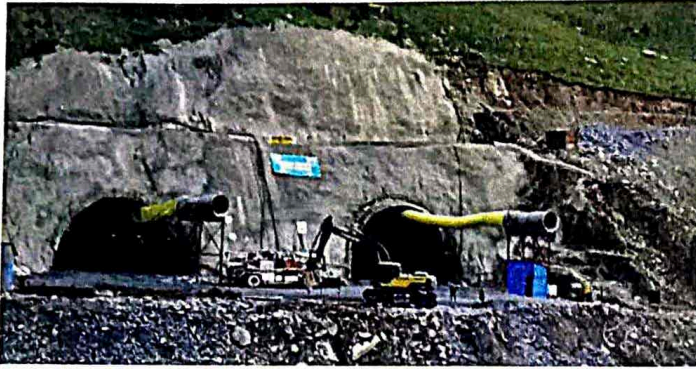
Construction Activity at Zojila Tunnel
